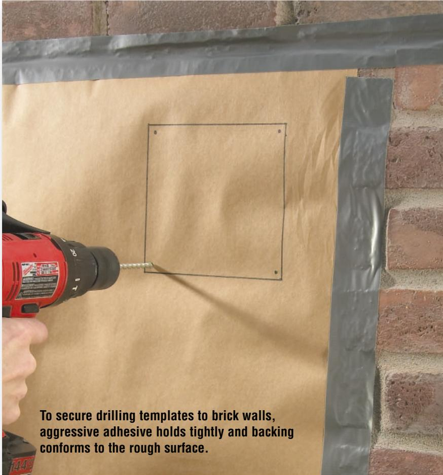
**To secure drilling templates to brick walls, aggressive adhesive holds tightly and backing conforms to the rough surface.**
